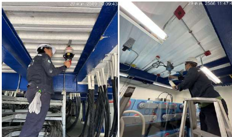
Fig.10 : Test all fire protection device at control building
