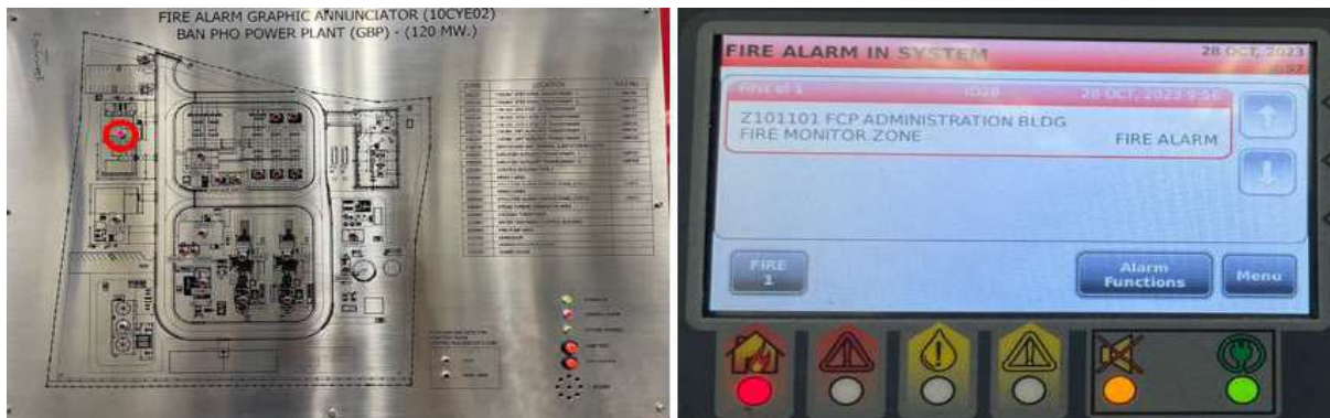
Fig.3: Fire alarm graphic and FCP in control room show alarm zone Admin building
