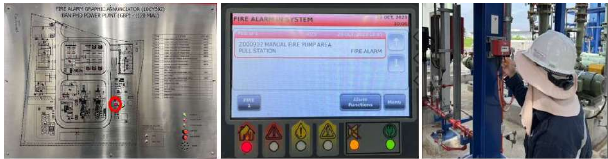
Fig.11 : Test manual call point at fire pump area
