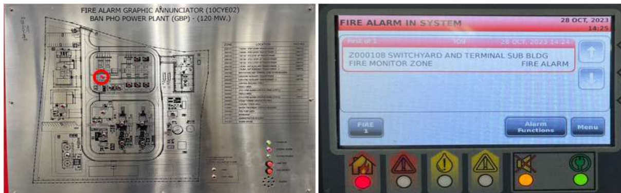
Fig.5: Fire alarm graphic and FCP in control room show alarm zone Switchyard and Terminal Substation building
