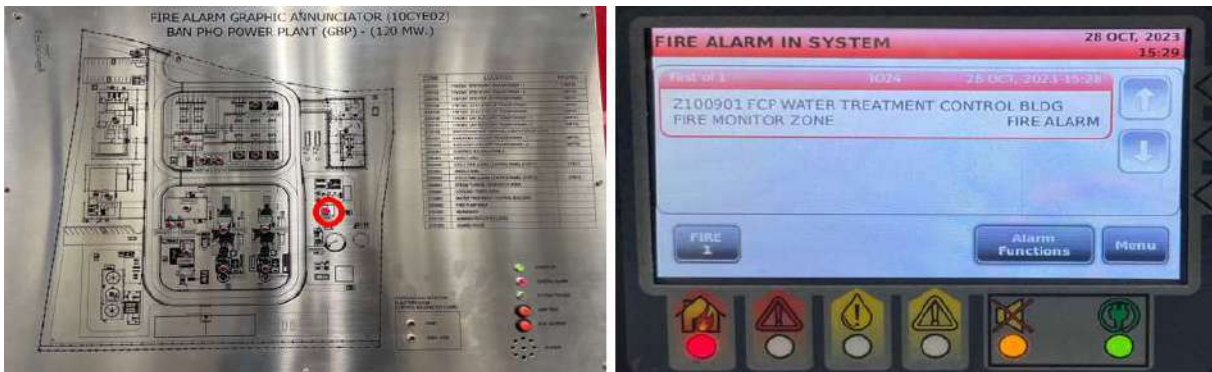
Fig.11 : Fire alarm graphic and FCP in control room show alarm zone water treatment building
