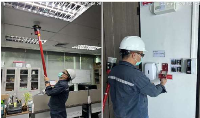
Fig.4: Test all fire protection device at Admin building
