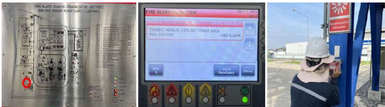
Fig.13 : Test manual call point at cooling tower area
