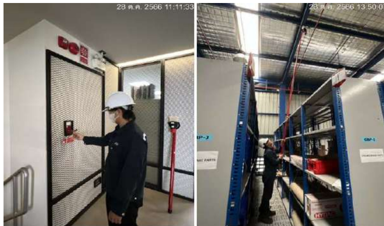
Fig.8: Test all fire protection device at workshop building
