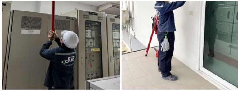
Fig.6: Test all fire protection device at Switchyard and Terminal Substation building
