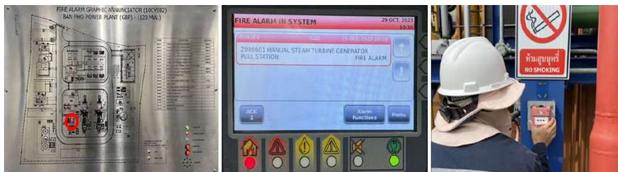
Fig.14 : Test manual call point at steam turbine area
