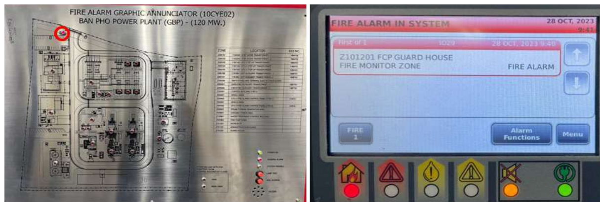
Fig.1: Fire alarm graphic and FCP in control room show alarm zone guard house
