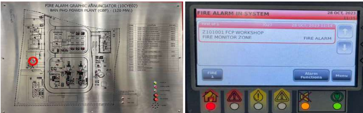
Fig.7: Fire alarm graphic and FCP in control room show alarm zone Workshop building
