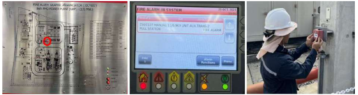
Fig.16 : Test manual call point at Unit aux transformer area
