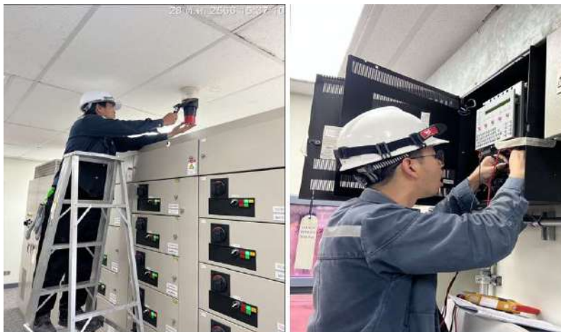
Fig.10 : Test all fire protection device at control building
